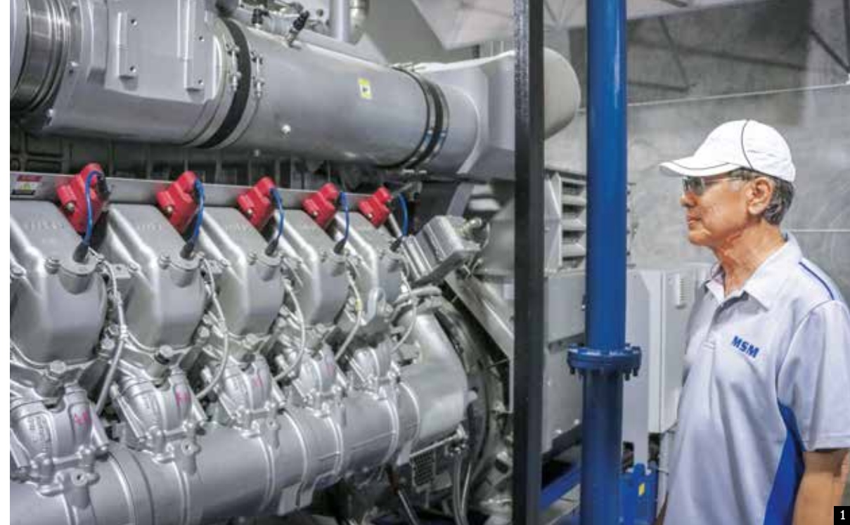
1 and 4 MTU Onsite Energy's combined heat and power plants enable GSL to save 160,000 euros a month in electricity costs. GSL also uses the waste heat to supply the cooling system with power. 2 Chainart Rakkaserm cultivates cassava tubers and supplies them to GSL. 3 The treated wastewater from the GLS cassava factory is used for irrigation on a reforestation project run by General Starch.
