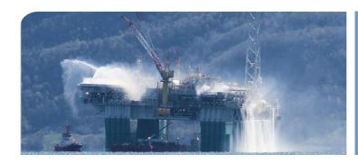
The fire extinguishing system is able to draw in over 4,000 liters of sea water a second for fire-fighting purposes.
