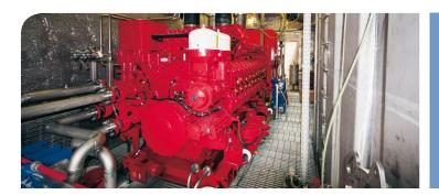
The pumps are driven by four MTU Series 4000 20-cylinder engines capable of 2.800 kilowatts each.
